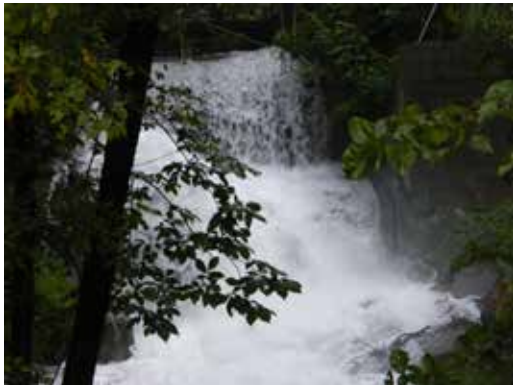
Gull Lake Dam after a ten-inch rainfall in 2008
